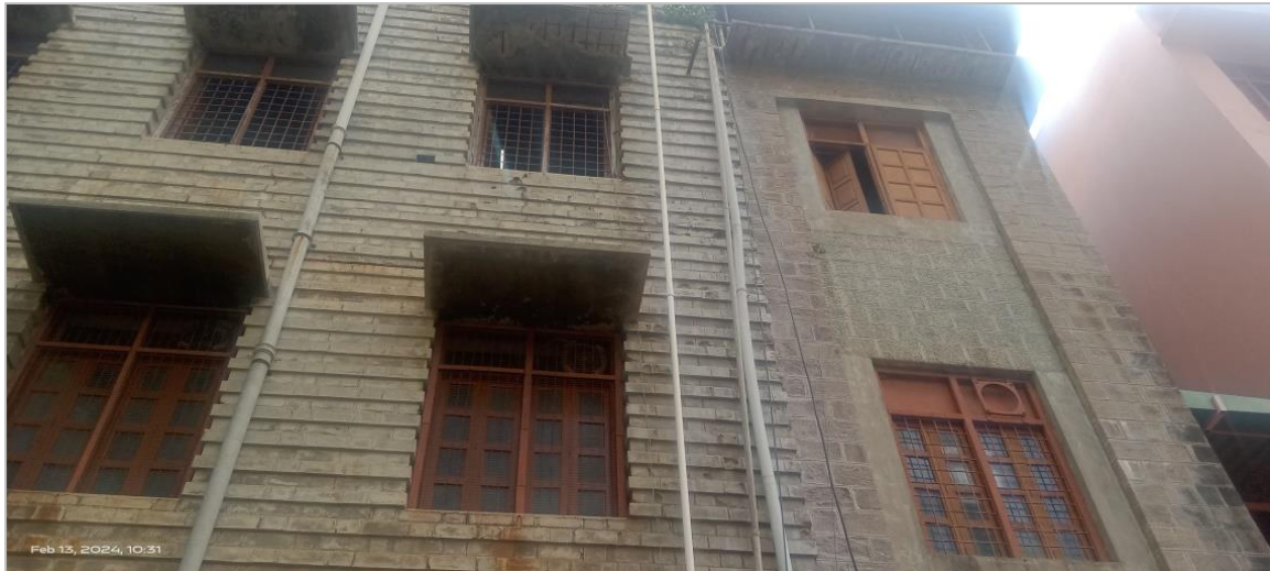
Plate 17: Rain water pipes
