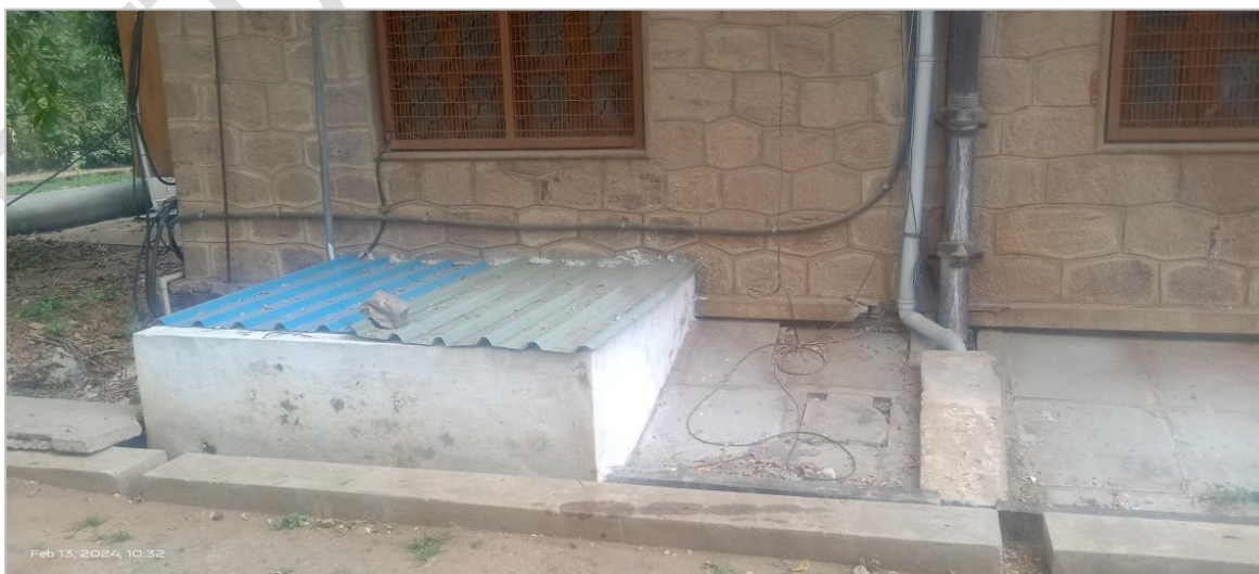
Plate 19: Dedicated rain water pits covered in tarpulin
