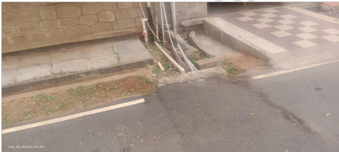
Plate 18: Rain water pipes connected underground
